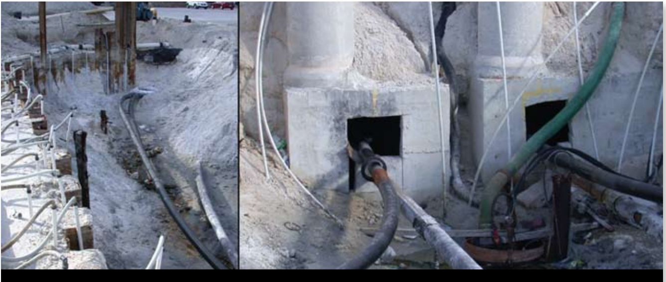
Because of the deep burial depth of the existing cable pipes into the newly installed HDD cable pipes, an extensive pit had to be excavated and fitted with an elaborate well-point system to keep the area and connected manhole relatively dry while pipe cutting and welding, as well as cable splicing, were completed.
