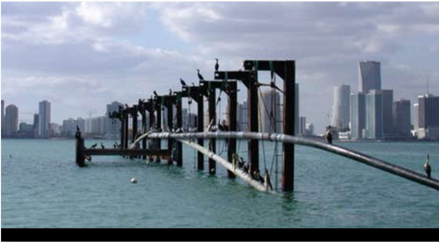
The existing cable pipes and newly installed cable pipes were brought above the water surface and aligned so that the pipes could be safely cut and the cables spliced.
